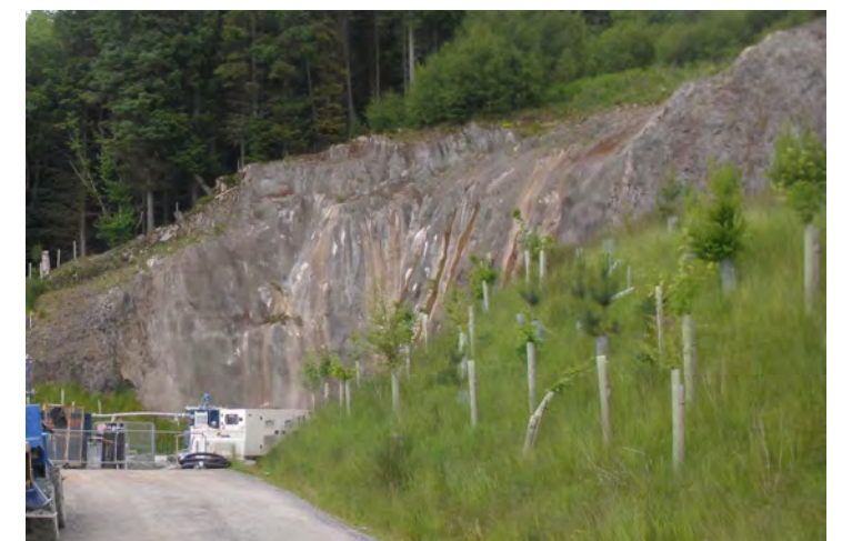
Examples of new landform created against cut rock face at Glendoe Tailrace
